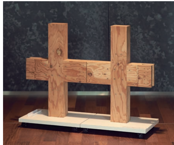
Model of Rigid Cross Joint
