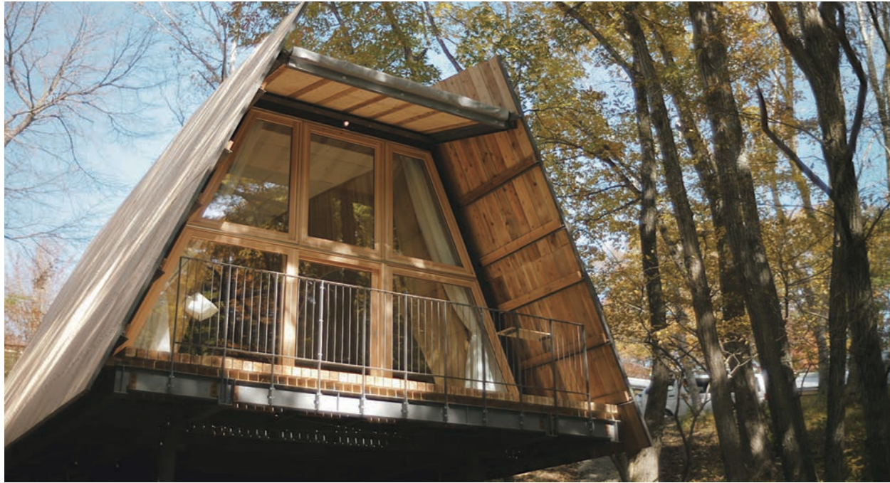
Exterior view of SANU CABIN (The cabins are arranged without tree logging as much as possible)
